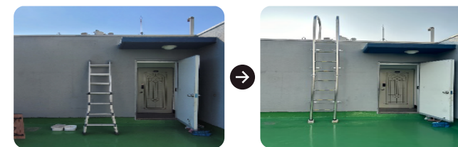
*Before and after installation of fixed ladders
