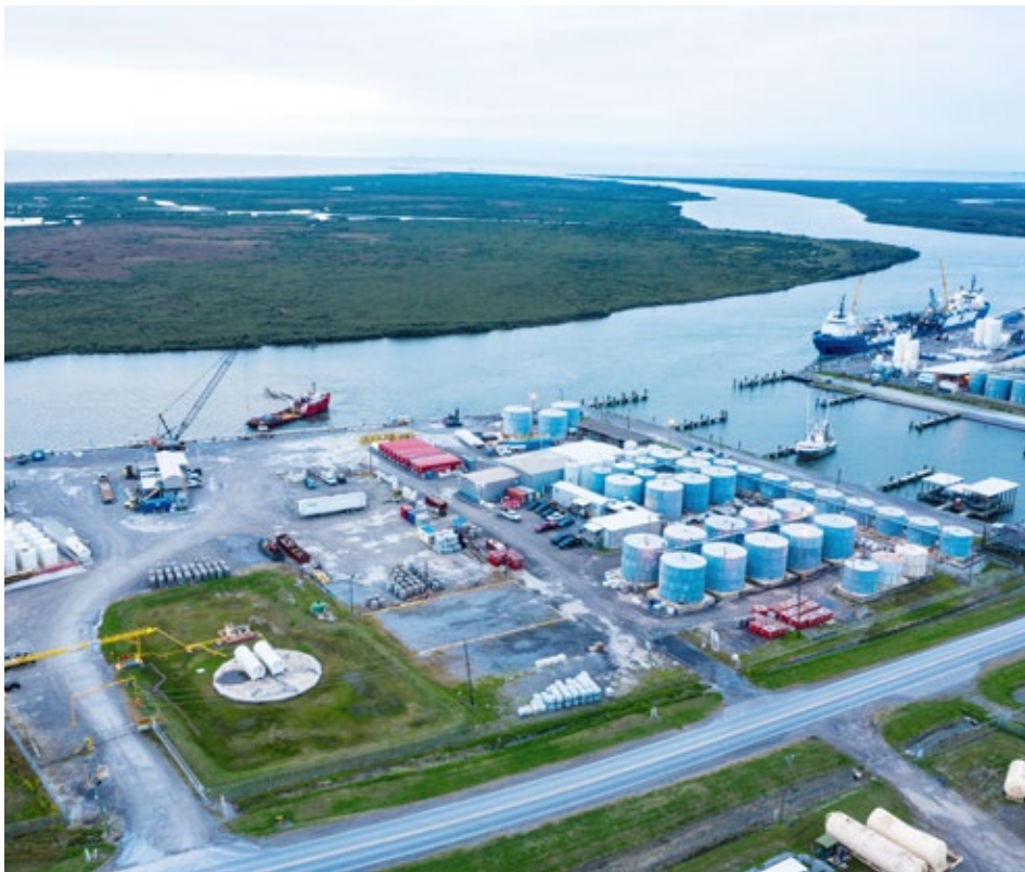
Aerial view of TETRA's full service 250,000 square foot fluids facility near Port Fourchon, Louisiana. One of the largest facilities on the Gulf Coast supporting deepwater operations in the Gulf of Mexico.
