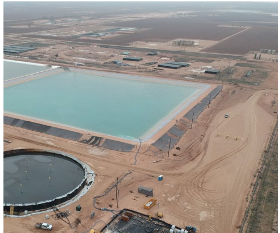
Aerial view of a treatment and recycling operation for a customer in the Permian Basin.
