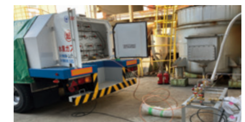
Hydrogen supply facilities used in the trial
