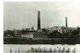
Amagasaki Boseki (Later, Dainippon Boseki) Head Office Plant
